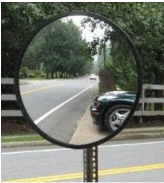
Figure 83: Convex mirror on the minor road to improve sight distance
