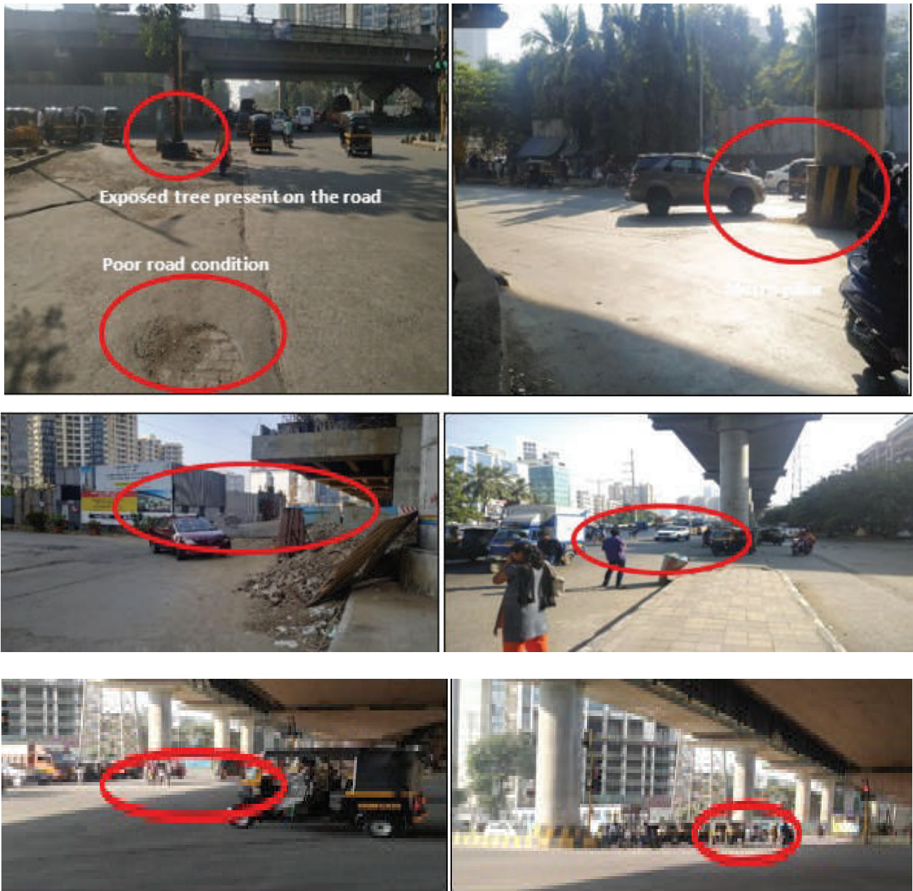
• Figure 40: Identified safety issues observed during the site visit at Magathane Depot Bridge Junction near Annex Mall
