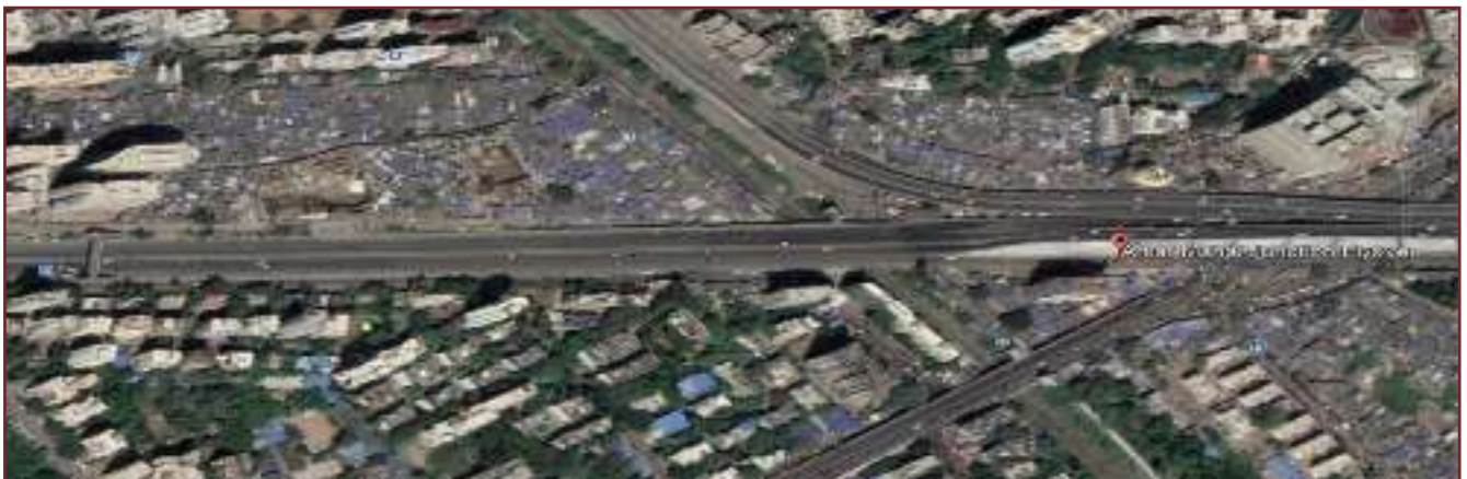
• Figure 47: Google earth view of Amar Mahal Junction, towards Thane, starting of Amar Mahal Bridge
