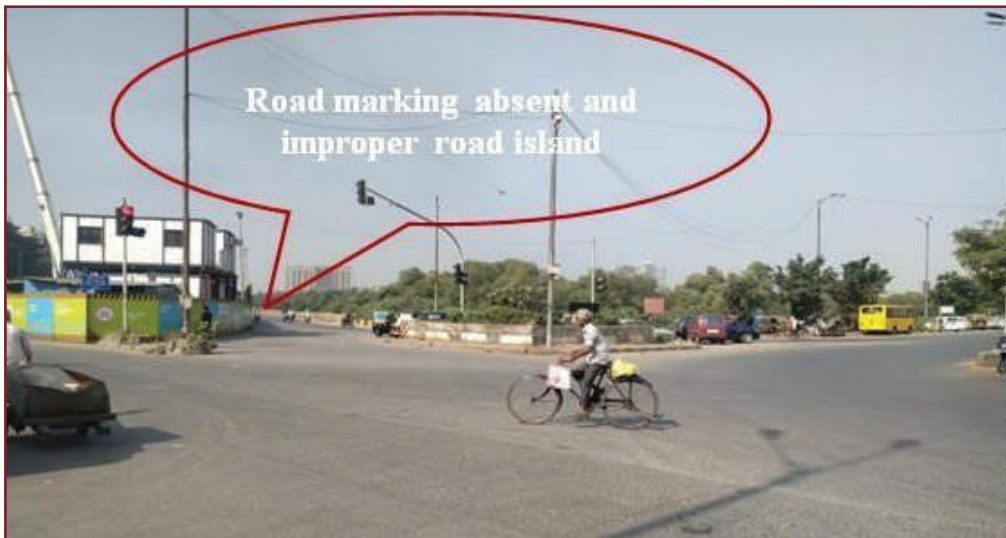
• Figure 29: Identified safety issues observed during the site visit at Y Junction, Sion Bandra Link Road, Dharavi
