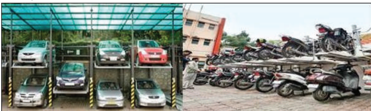
Figure 113: Prefabricated automated multi-level parking
