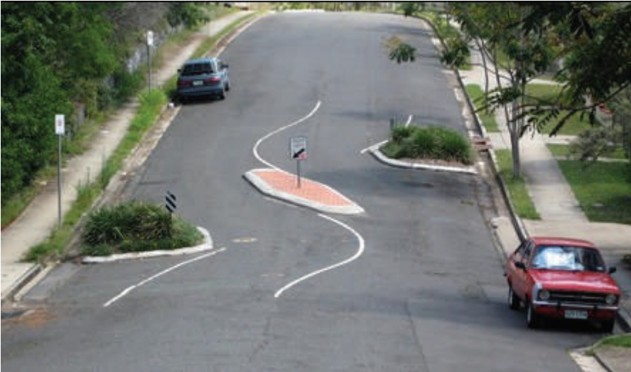
Figure 80: Staggering in two lanes by providing chicanes
