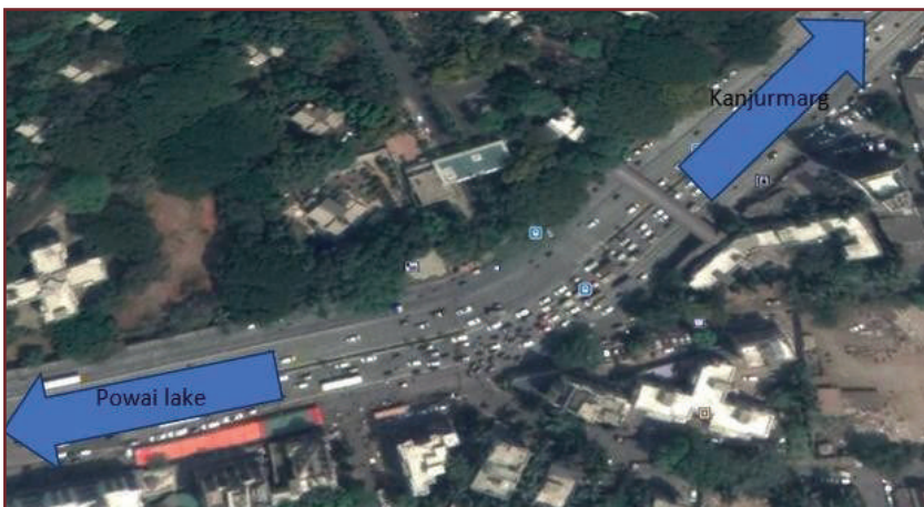
• Figure 56: Google earth view of opposite IIT Bombay main gate, IIT Bombay Signal, Powai
