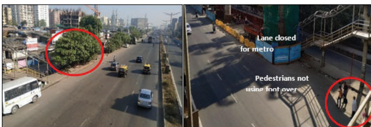
• Figure 49: Identified safety issues observed during the site visit at Amar Mahal Junction, Towards Thane, Starting of Amar Mahal Bridge
