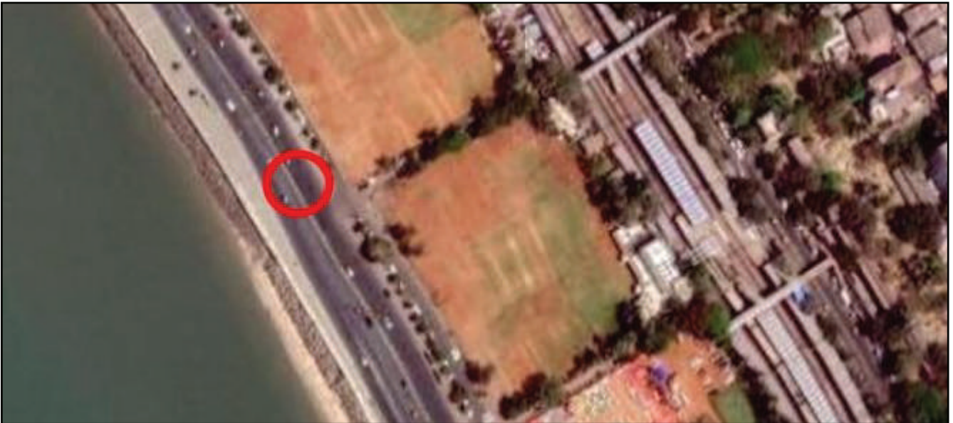
• Figure 21: Google earth view of Megdoot Bridge, opposite Islam Gymkhana, N.S. Road
