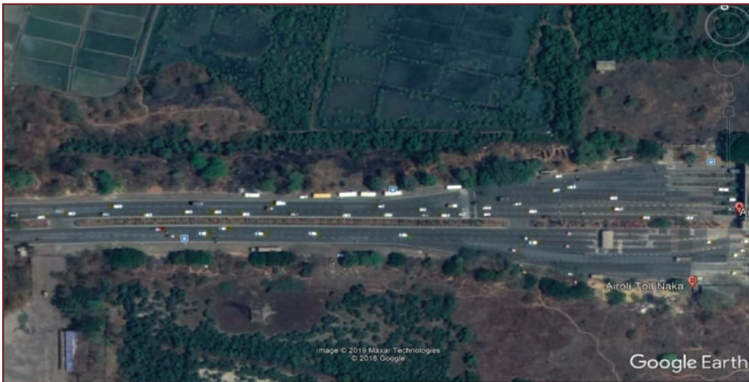
• Figure 53: Google earth view of Airoli Toll Naka, before Airoli Bridge, Thane-Mumbai Way, Airoli Mulund Way
