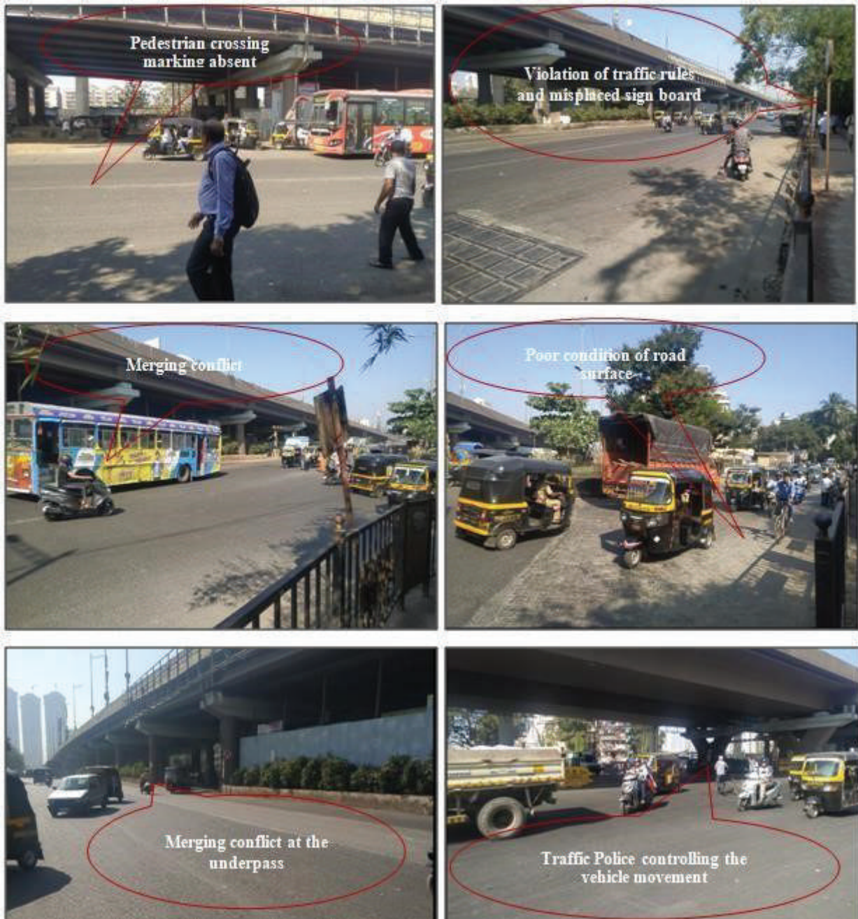
• Figure 38: Identified safety issues observed during the site visit at Sanjay Gandhi National Park Gate, Under Flyover, Borivali East
