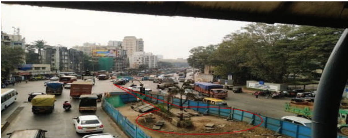
• Figure 58: Identified safety issues observed during the site visit at location opposite to IIT Bombay main gate, IIT Bombay Signal, Powai
