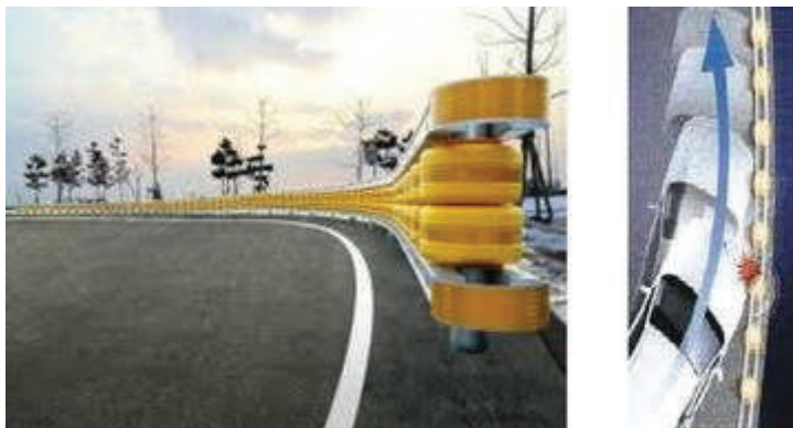
Figure 84: Rolling Barriers at the roadside and vehicle collision
