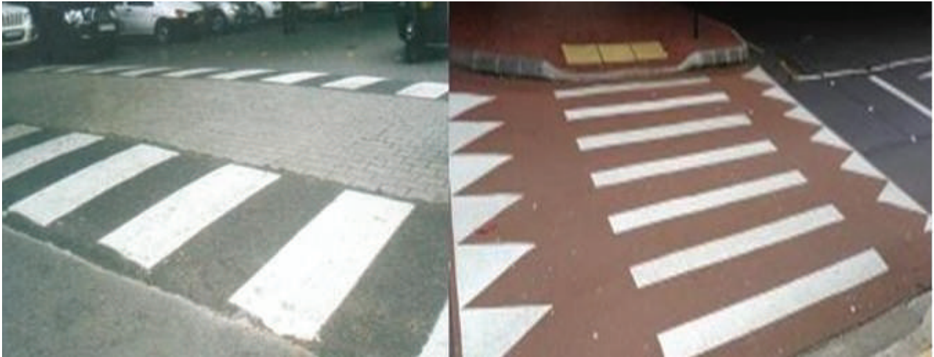
Figure 73: Speed tables or raised pedestrian crossing
