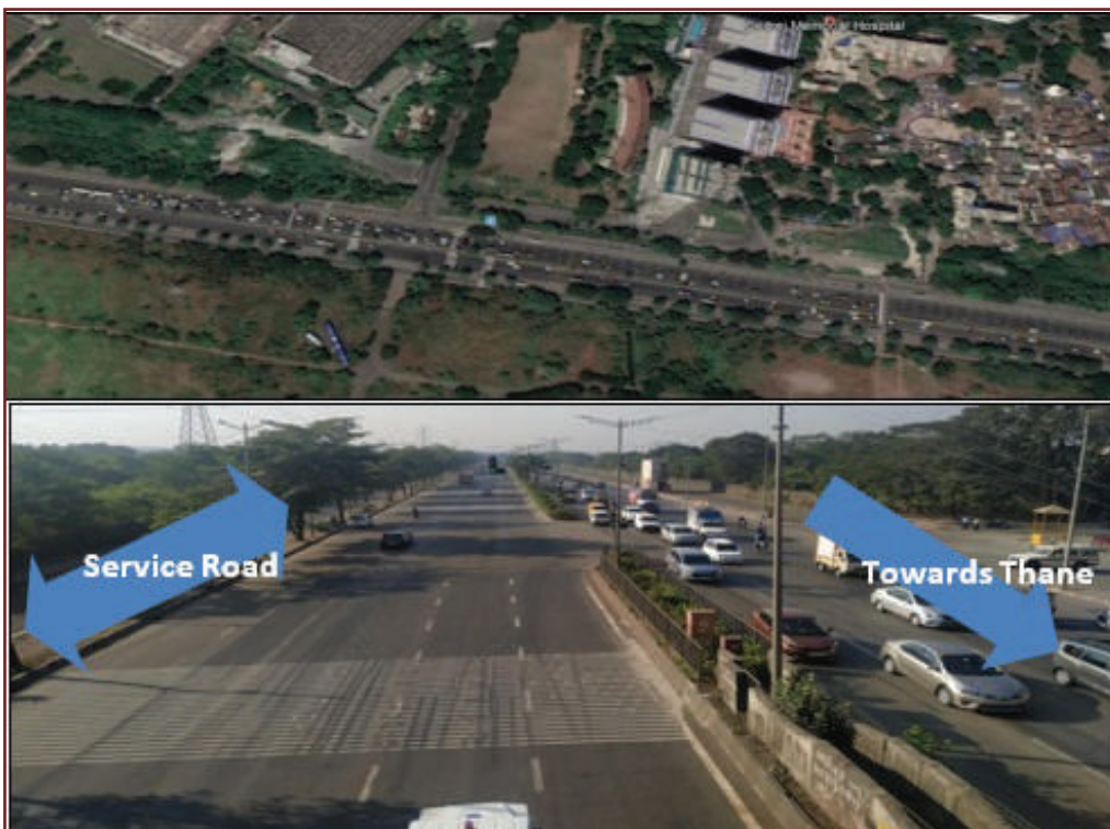
• Figure 50: Google earth view and photograph of Godrej Ghoda Gate Signal, Vikhroli (East)
