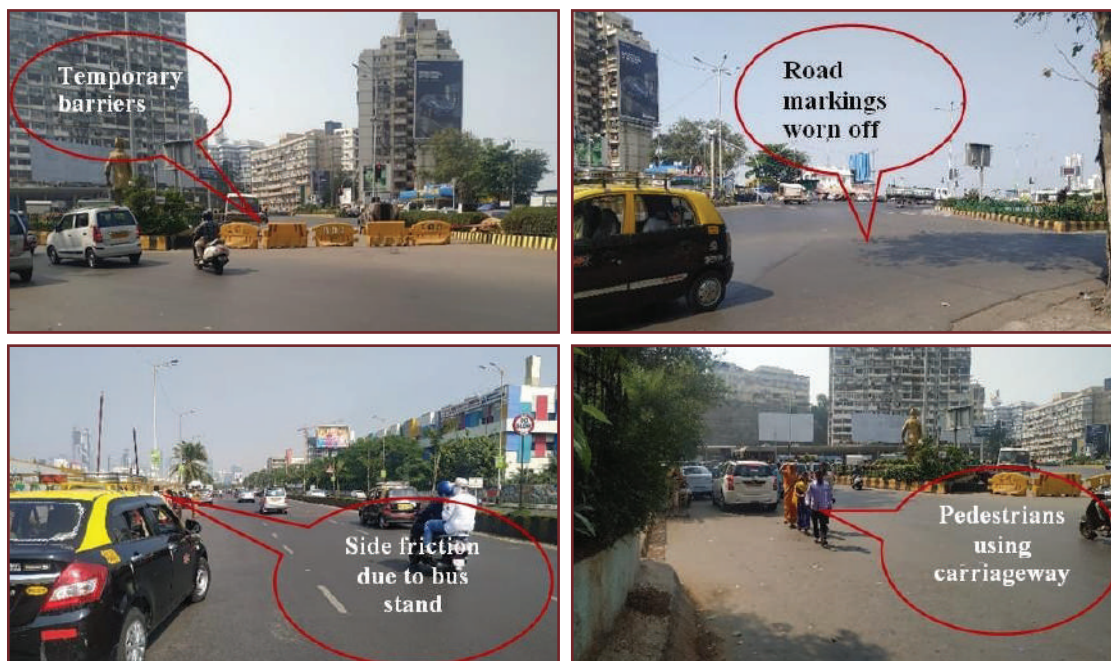
• Figure 11: Identified safety issues observed during the site visit at Haji Ali Junction
