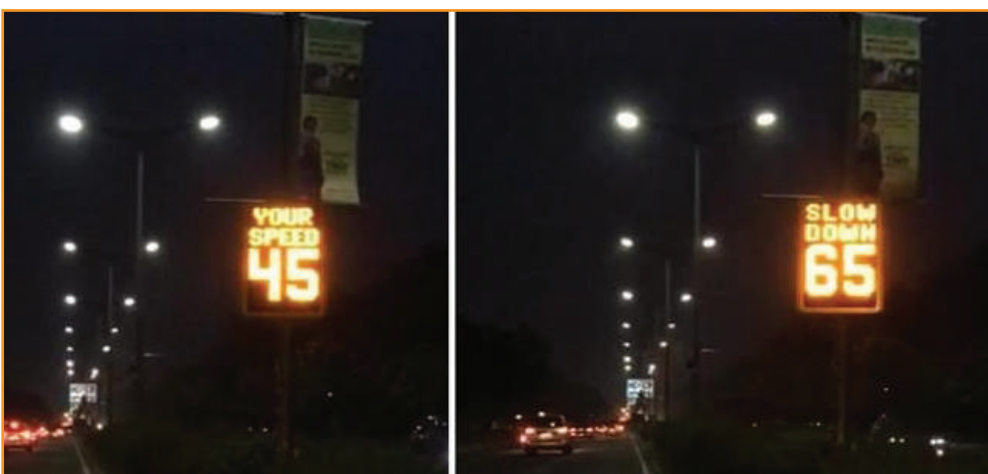
Figure 71: Driver Feedback Sign displaying vehicle speeds
