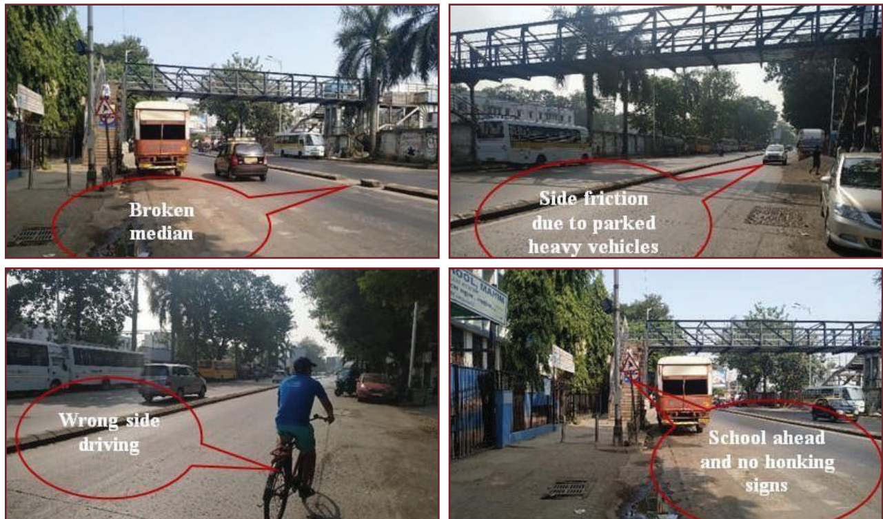
• Figure 20: Identified safety issues observed during the site visit Near Mahim Phatak, Senapati Bapat Road, Mahim
