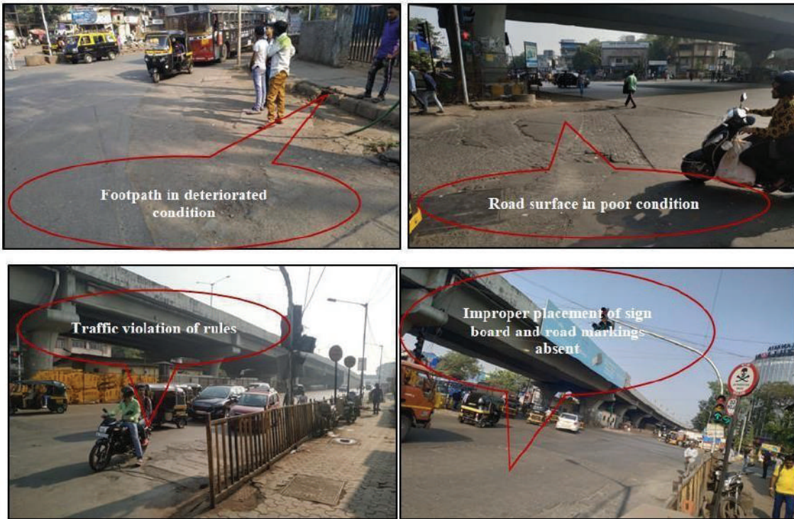
• Figure 32: Identified safety issues observed during the site visit at CST Bridge, Kurla West
